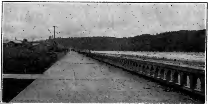
NEW CONCRETE PROMENADE AND SEA-WALL, SEASIDE, ORE.
